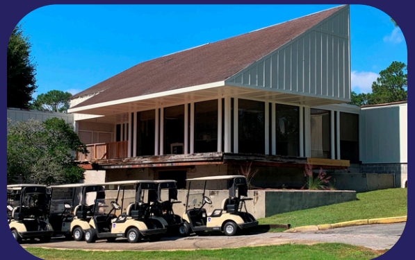
The decorative wing on the back of the building will have new architectural shingles.
