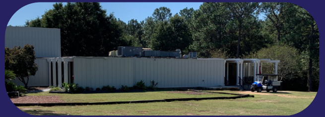
The flat surface of the clubhouse roof will be coated with 60-mil PVC
